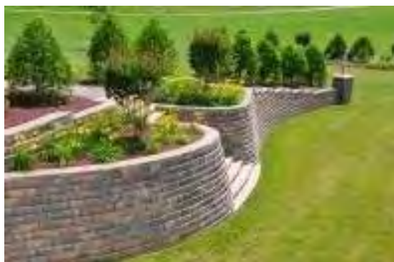
Anchor Highland Wall - Bull Run
